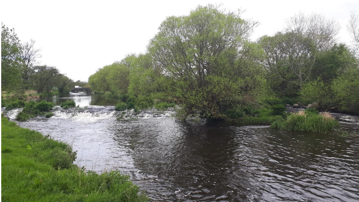
Figure 2 Weir downstream of St Johns Bridge at Toberona, Dundalk on the Castletown_030
