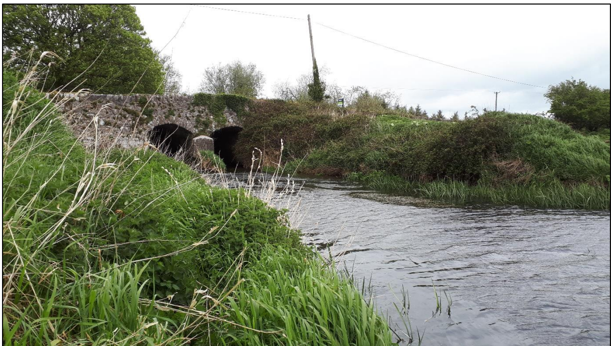
Photograph of WFD operational monitoring point at Annagh Bridge, taken on 26 th of April 2019
