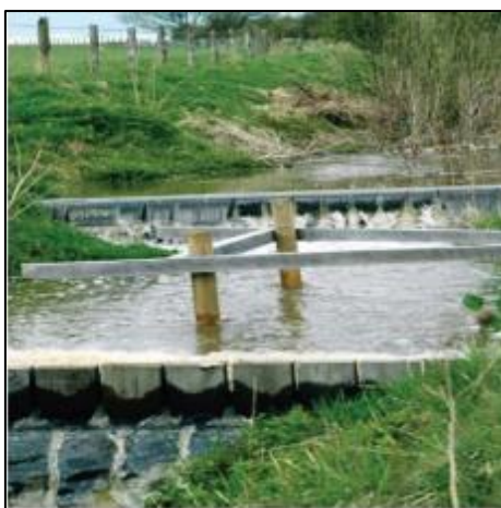
Figure 5-5 Leaky barrier installed in a farm ditch (Quinn et. at., 2007).
