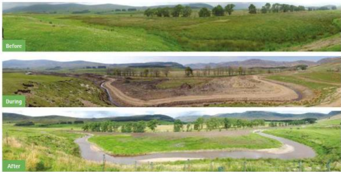
Figure 5-10 Remeandering carried out by the Esk Rivers and Fisheries Trust on the Rottal Burn (South Esk) (Source: SEPA (before and during) and Kenny MacDougall/Fraser Murdoch (after), amended for SEPA Natural Flood Management Handbook – See the River Restoration C
