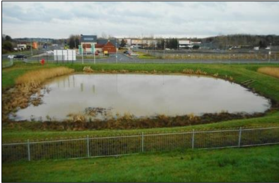
Figure 5-4 A sustainable drainage system (SUDS) pond beside the new Glenmill housing development at Darnley Mains, UK ( https://www.geograph.org.uk/photo/5274370 )
