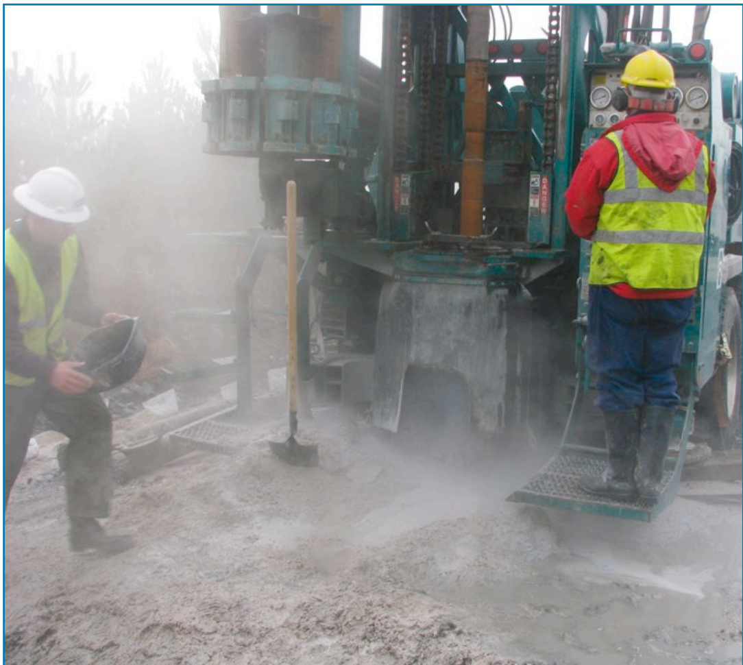
Installation of a monitoring well in Galway.
