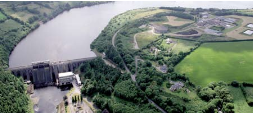
Reservoir development along the Lee was carried out between 1953 and 1957. Two dams were constructed, the photo above is of Inniscarra. The dam is 21.3 meters high and the reservoir behind it is 9km 2 in size. It is one of 15 large dams in Ireland. It's original purpose was for the generation of electricity. Now the impounded water is the most important water scheme in the South Western district. Inniscarra Lake is used for water sports including rowing and water skiing.
