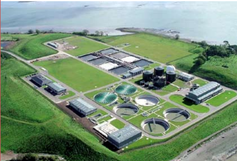
Carrigrennan waste water treatment plant serves Cork City, Tramore Valley, Glounthaune, Glanmire and Little Island. It can treat the effluent equivalent to a population of 413,000. It has been effective in improving the quality of water in the river Lee and its estuary since the plant became operational in 2004.
