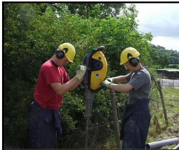
Plate 1. Installation of piezometers.
