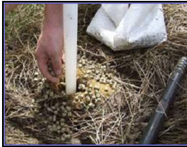
Plate 2. Piezometer at surface showing borehole packed with bentonite.
