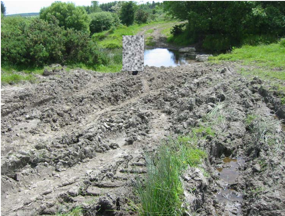
Plate 3.3 A view of the ford at Reanagullee (Grid Ref X 21817 86760). The damage caused by passage of heavy machinery is visible in the foreground.
