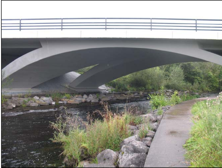
Plate 3.1 N15 Bridge over River Eske
