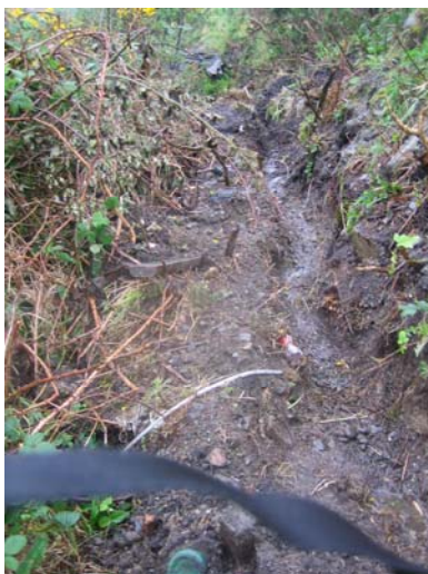
Figure 4.14 Silt run-off to channel at RHAT 9
