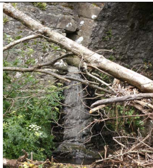
Plate 4.8 Greyish coloured discharge from sewage outfall at Clonea Bridge, plus tree debris in the foreground
