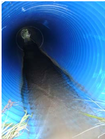
Plate 3.1 Site 8 Photo 1 (See Figure 3.6 for overview of location)
