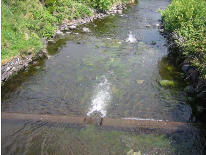
Plate 3.5 Existing weir at the outlet from Glenbeg Lough into Ownagappul River
