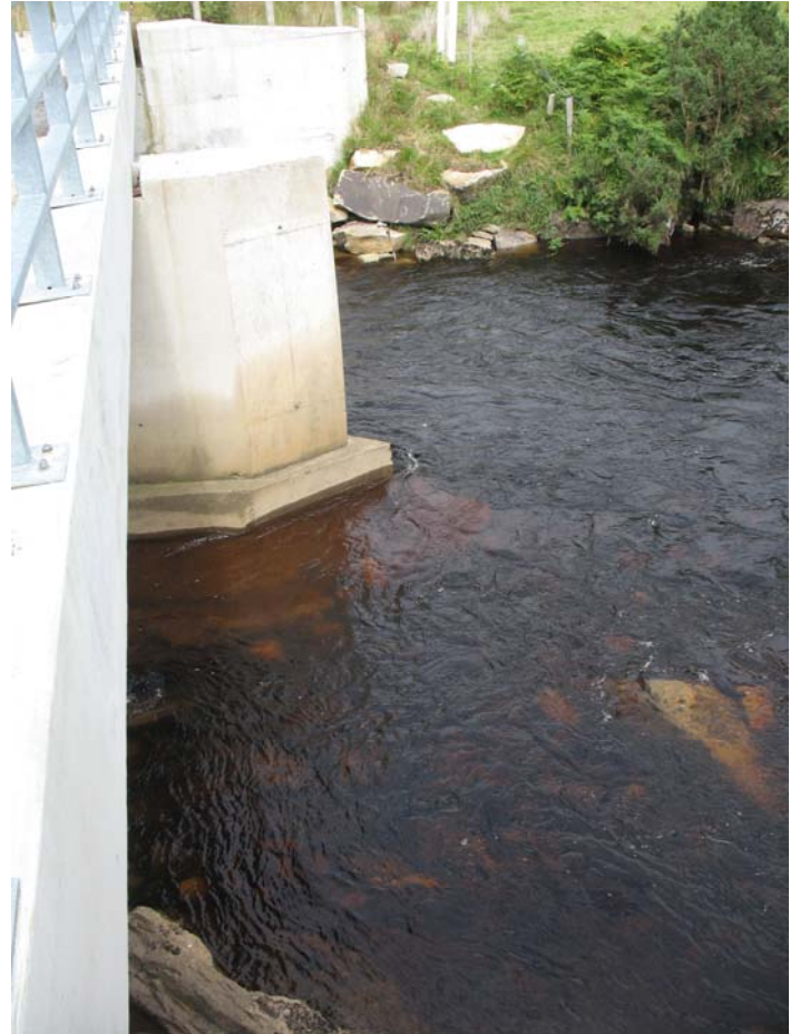
Plate 3.3 Large central pier embedded in concrete
