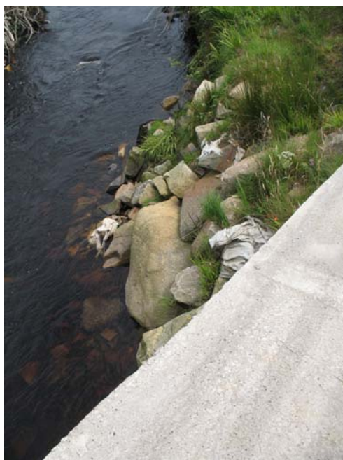
Plate 3.4 Rock armouring upstream and downstream of the bridge
