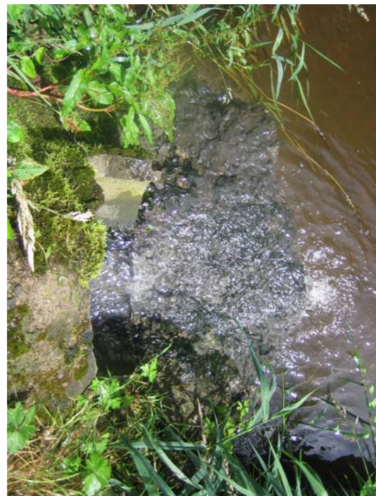
Plate 3.15 outfall from Glanbia which discharges directly into the Nore main channel
