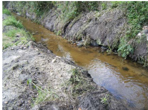
Plate 3.2 In-Channel and bank clearance works on the Glasheroge Stream
