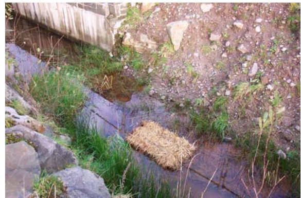
Plate 3.9 Iron precipitate in drain at construction site. Photo by Dr Julie Fossitt
