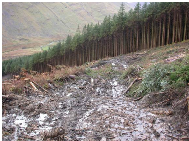
Plate 3.4 Forest track with damaged brash mat and significant flows of surface water.
