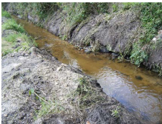
Plate 3.3 In-Channel and bank clearance works on the Glasheroge Stream
