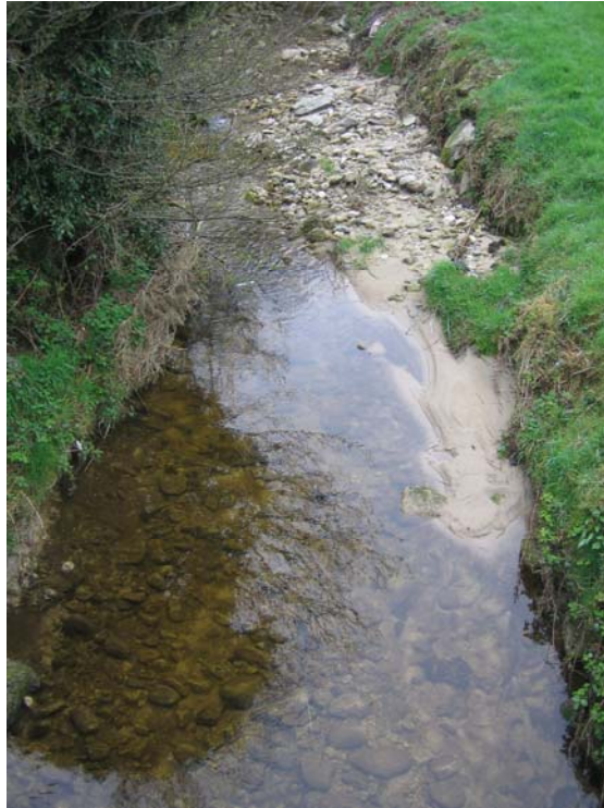
Plate 3.5 Increased levels of silt in-channel downstream of works
