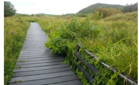
BOARDWALK INSTALLED AT FENOR BOG
