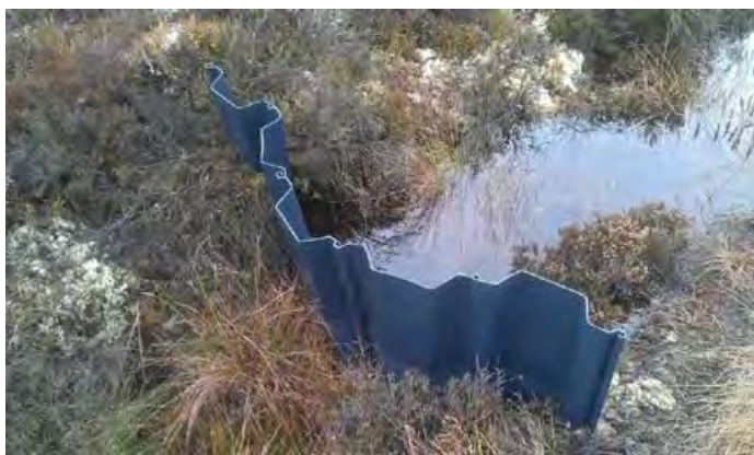
Figure 2: Within five years blocked drains revegetate with peat-forming vegetation including Sphagnum moss as seen in this drain on Lodge Bog in Co. Kildare. Photo: IPCC.
