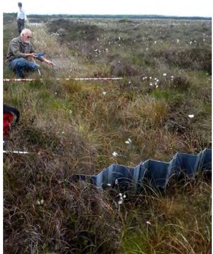
Figure 1: A Geoflex plastic dam constructed in a bog. Within hours the water backs up behind the dam. A raised water table on a bog works to maintain the carbon store contained within the peat soil of the bog. Photo: IPCC.
