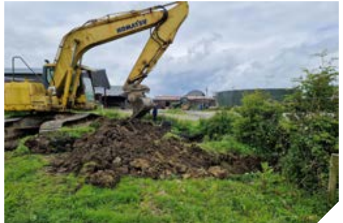
The willow bed is prepared by digging out an area 4 metres wide to allow for the sowing of the stems.
