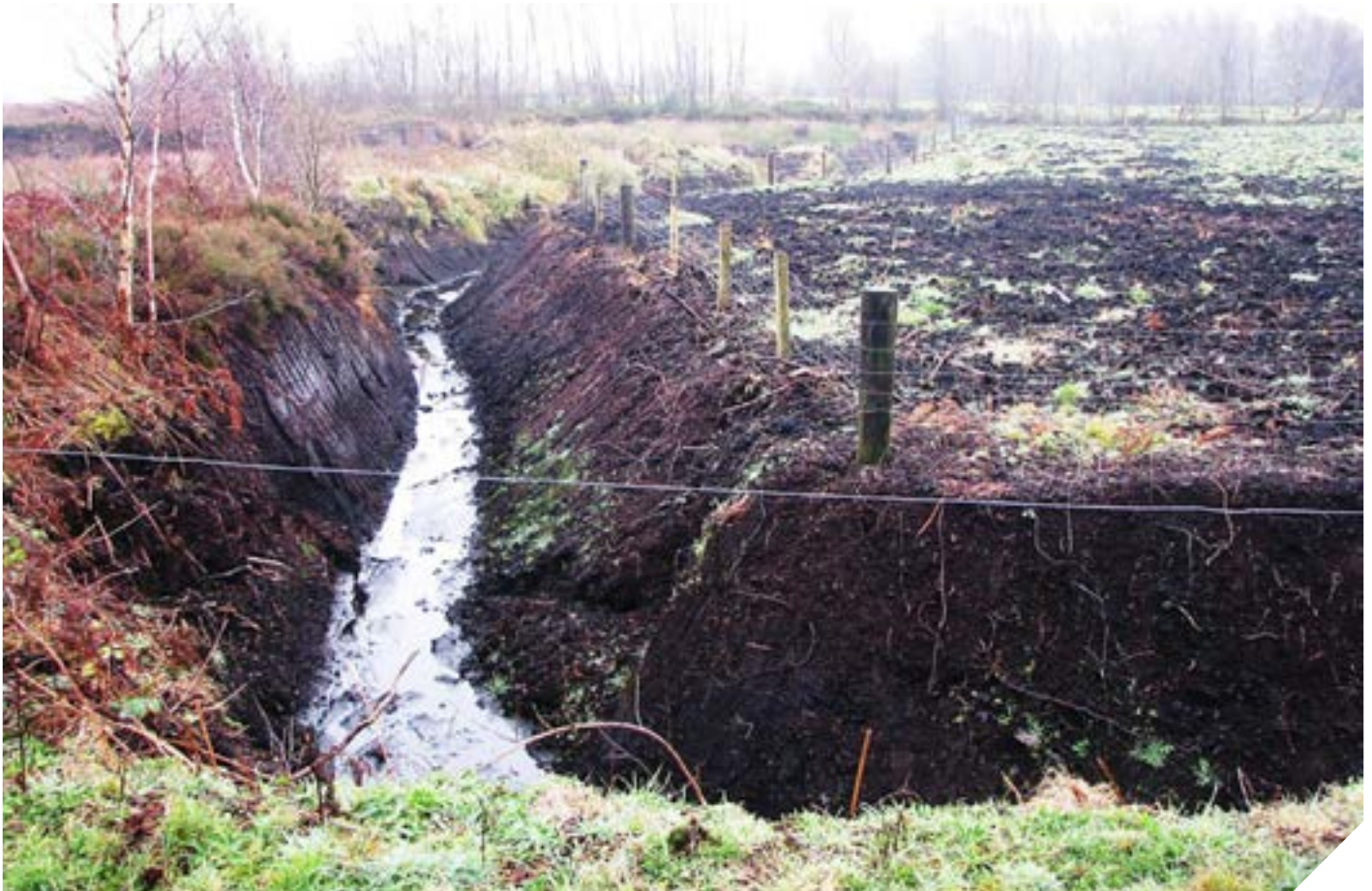
Photo 1 shows a typical scenario where drainage channels in and alongside peatlands are usually >0.5 m and often >1 m deep.
