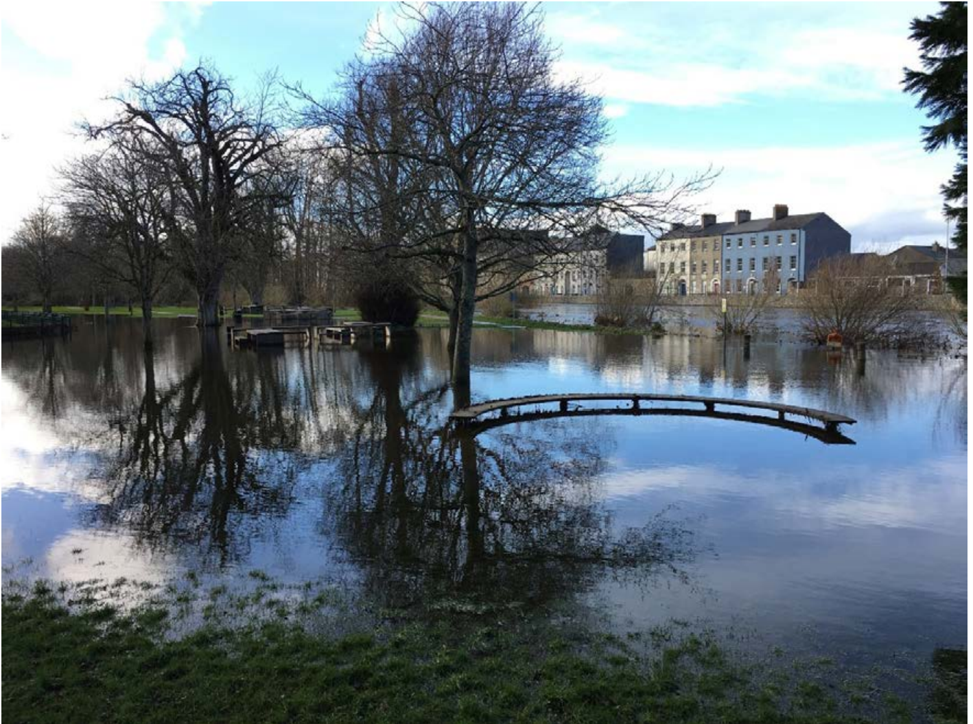
Making space for water. Dennis Burke park in Clonmel floods in February 2021. By working with nature, the park serves multiple functions including supporting amenity, biodiversity, alleviating flood risk and providing essential services in Clonmel with greater climate resilience.
