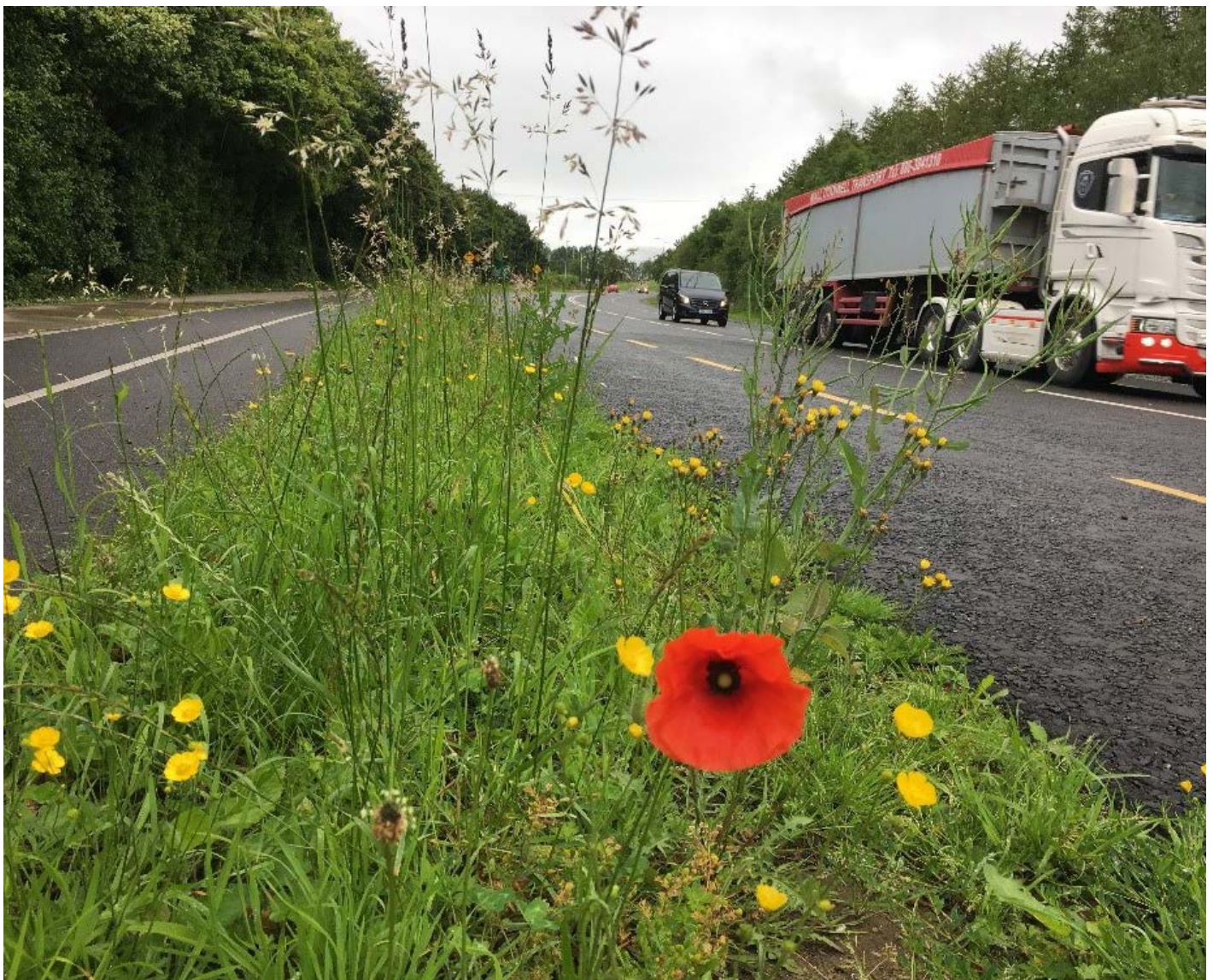
Filter strip on N24 provides not only extra surface run off soakage but also biodiversity and amenity benefits.
